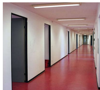
Renovated hallway at Takustraße 6
